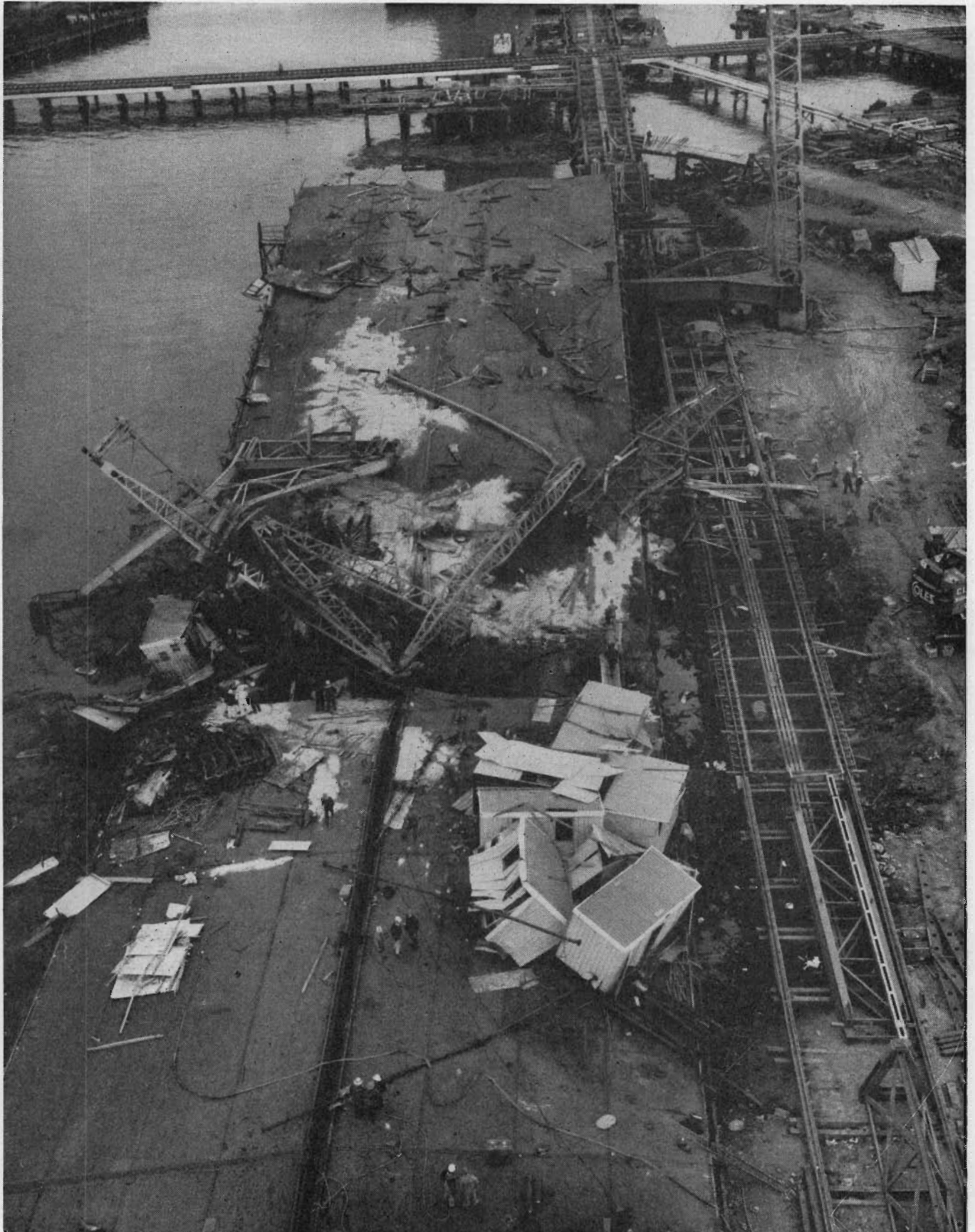
PLATE 1. VIEW OF COLLAPSED SPAN FROM TOP OF PIER 10.
